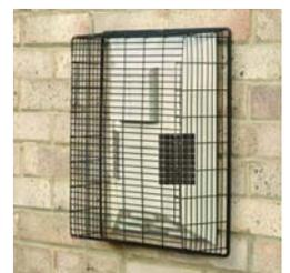
Recessed rear vent terminal (for use if external space is restricted)
